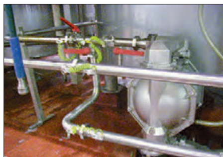
3" sanitary pump used to transfer cosmetic basis for shampoos
